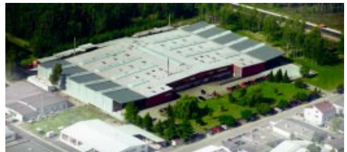
Werk in Speyer / Deutschland Production facilities in Speyer / Germany
